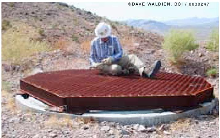
A grate is placed on a vertical culvert to maintain airflow in the mine.
