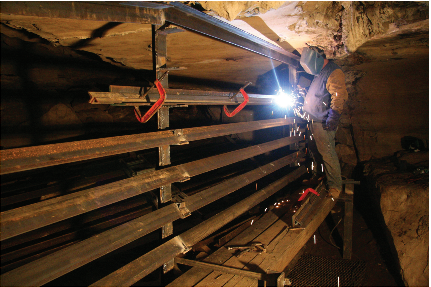
Figure 4. Constructing an angle-iron bat gate, with stiffeners. Photo © Jim Kennedy, BCI.
