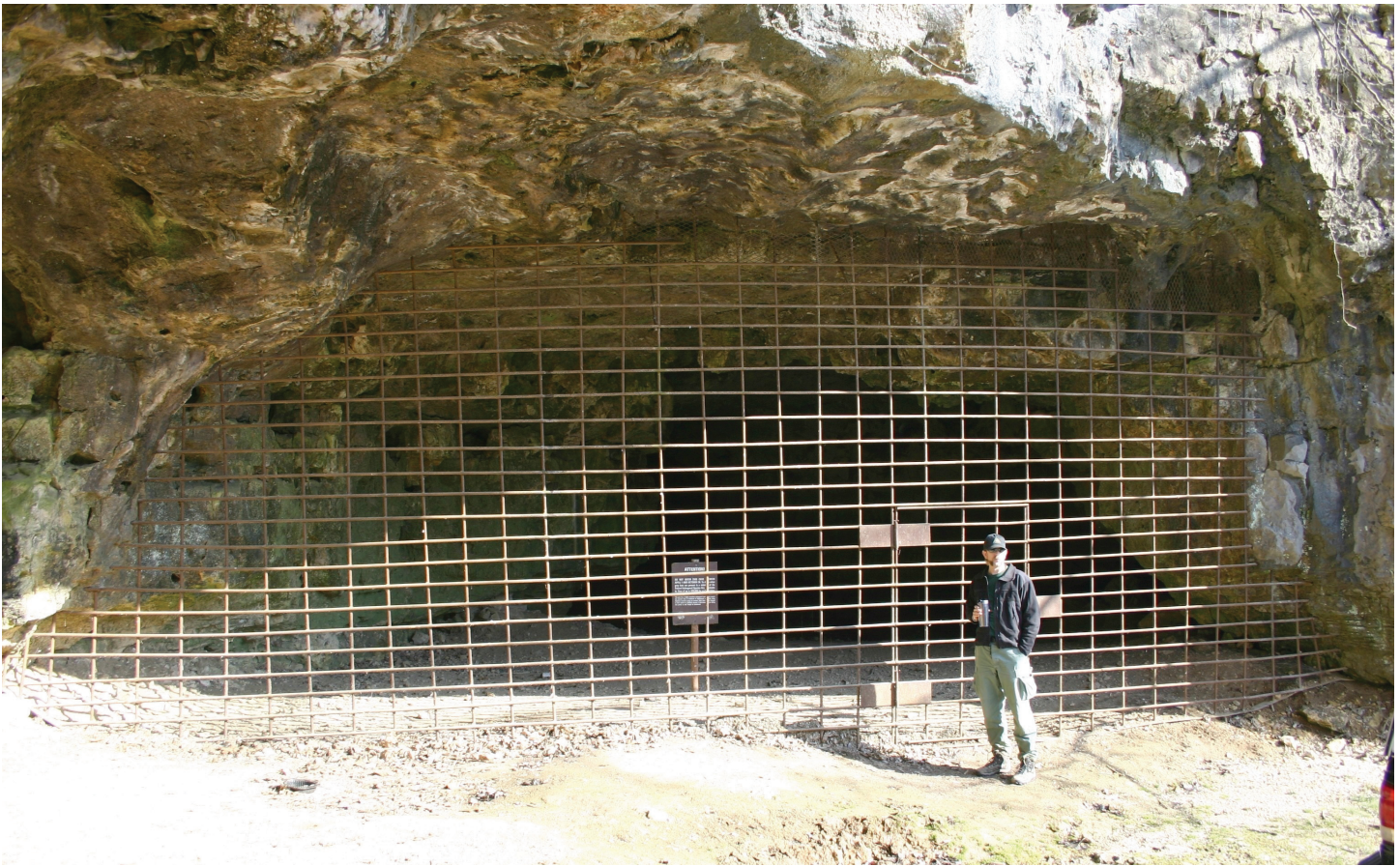
Figure 2. Rebar gate on gray bat maternity cave. Note closely spaced vertical supports. This cave was abandoned by the bats shortly after the gate was installed. It has since been replaced with a more bat-friendly design. Photo by Bill Elliott.
