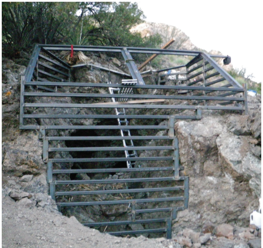
Figure 3. Rectangular tube steel gate on an abandoned mine in Arizona. Photo by Jerry Fant.
