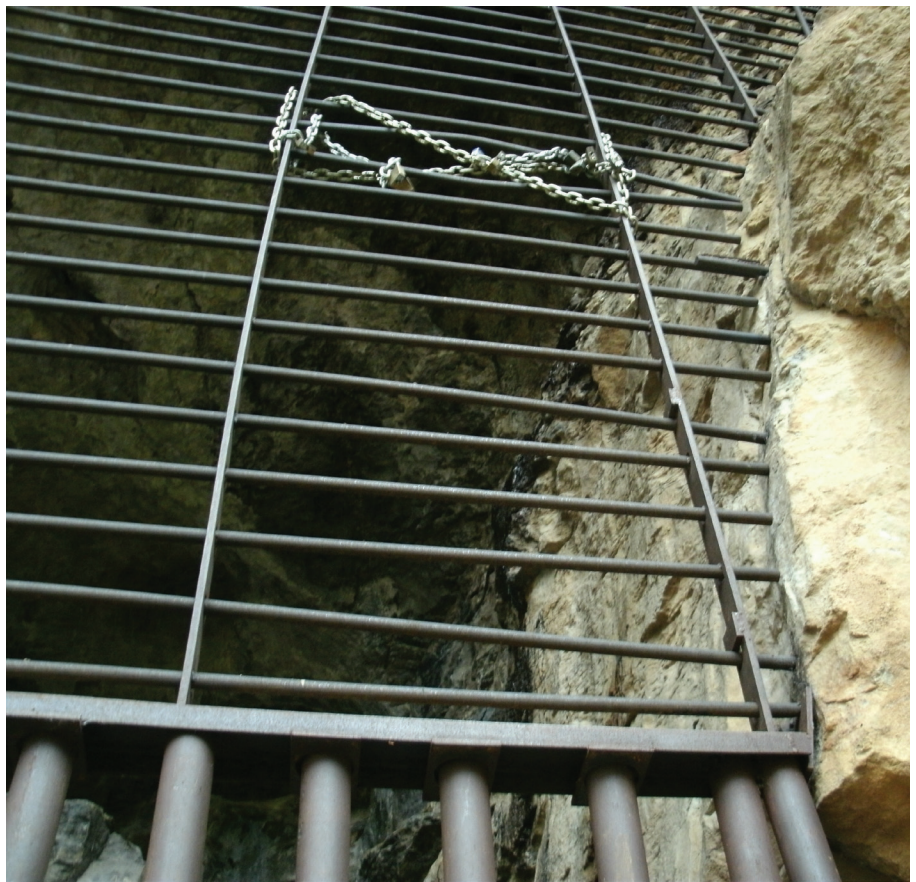
Figure 5. Mangalloy cave gate in Utah. Note how bars have been bent to illegally gain access, necessitating temporary repairs. Photos © Jim Kennedy, BCI.
