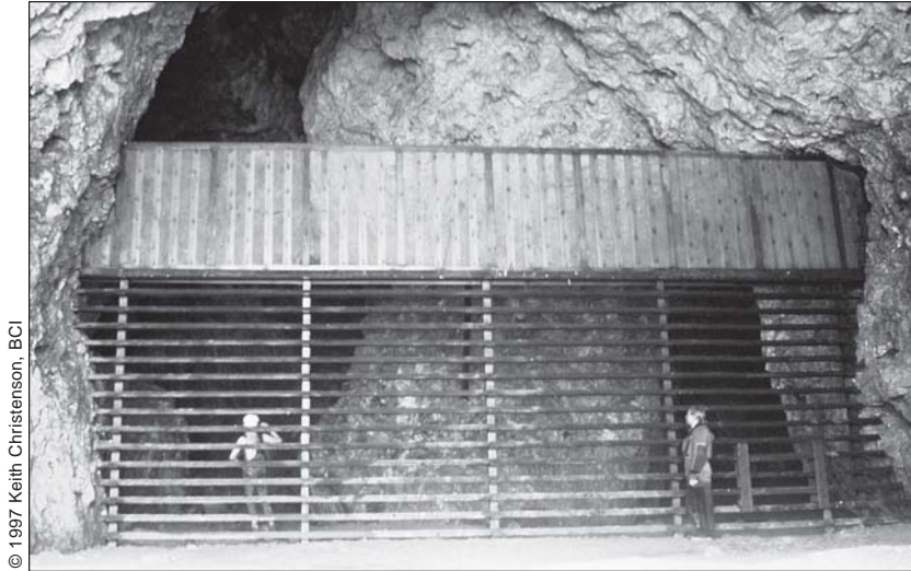
Figure 9. Half or “flyover” gate. Note the removable bar at bottom right. Expanded metal mesh covers the overhanging top portion, making it extremely difficult to climb over. Coating the overhang with grease also helps repel trespassers.
