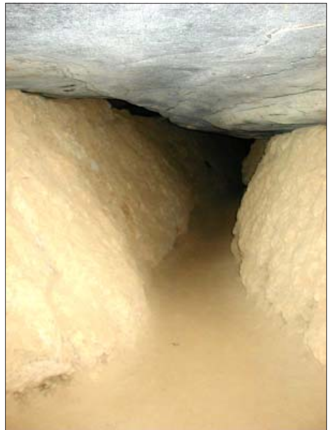
Figure 7. Heavily modified tourist trail in Saltpetre Cave. Original fossil stream passage is approximately 10m (33 feet) wide and up to 0.4m (1.3 feet) high. Current dimensions of the tourist trail are approximately 1.7m (5.5 feet) high by 1.2m (4 feet) wide, with excavation spoil piled to the sides of the tourist trail blocking access to the remaining original passage. Photo by Jim Kennedy, © 2000.
