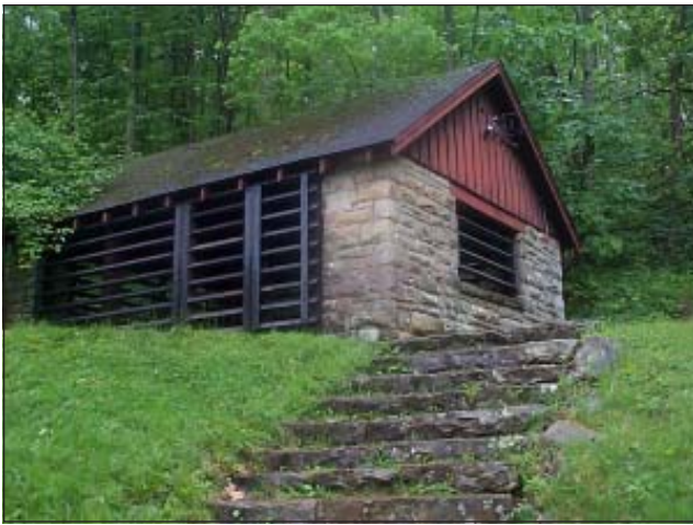
Figure 8. Building over Main Entrance to Saltpetre Cave after restoration work. Note bat-friendly horizontal bar gates. Photo by Traci Wethington, © 2003.
