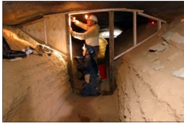
Figure 9. Caver volunteers Dale Lofland and Tanya McLaughlin constructing the temporary wooden wall for air flow diversion along a tourist route in Saltpetre Cave. Location is approximately same as in Figure 7. Photo by Jim Kennedy, © 2003.
