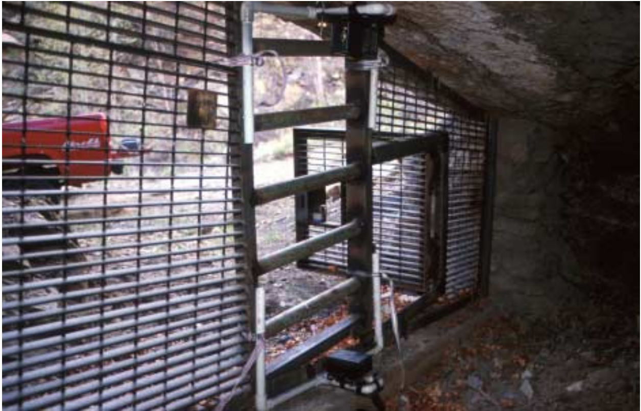
Gate installed in Colorado at a mine that supports a colony of Townsend's big-eared bats. (Photograph credit Kirk W. Navo, Colorado Division of Wildlife, Monte Vista, Colorado).
