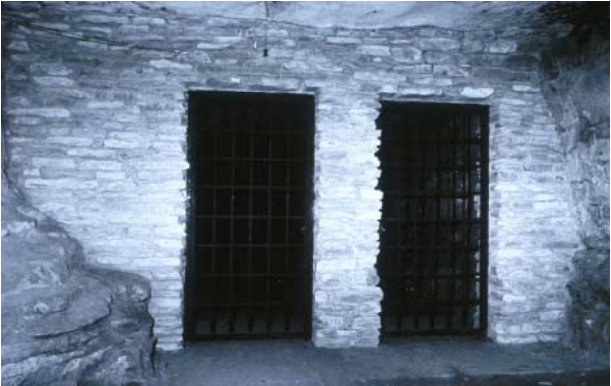
Early stone wall and gates constructed at Wyandotte Cave, Indiana. This structure severely restricted airflow and bat movement and contributed to a drastic decline in Wyandotte Cave's hibernating Indiana bat population. (Photograph Credit Virgil Brack, Environmental Solutions and Innovations, Cincinnati, Ohio).
