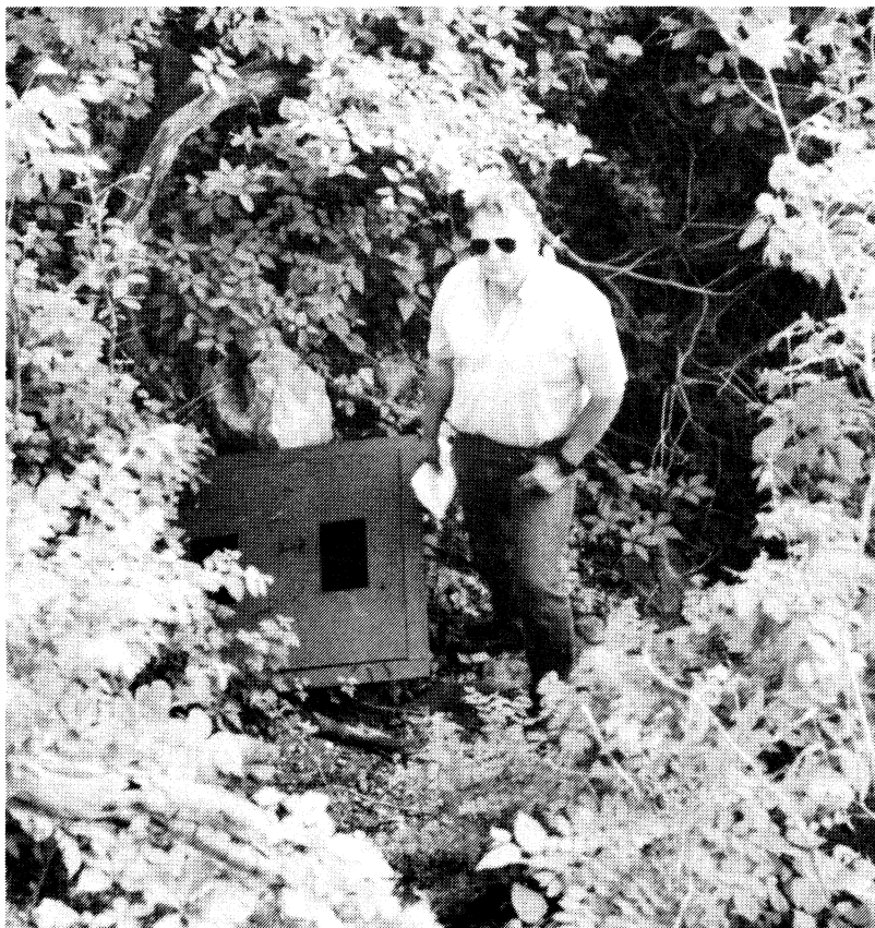
Bob Taylor stands beside the gate at Lon Odell Memorial Cave in Dade County. The gate is atop a 14-foot culvert with welded steps over a 40-foot drop to a talus cone floor. Note the 6" x 10" holes for use by pipistrelle bats. The gate protects prehistoric human footprints and torch remains found in the cave. The door to the gate was manufactured by Don Rimbach and Earl Hancock.
