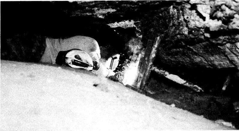
The gating of Fourteen Forty Cave in Wright County in 1995 by Ozark Highlands Grotto nears completion. David Binns uses a portable welder fueled by a portable generator (both located outside of the cave to prevent hazardous fumes from doing harm to the welder and cave lifeforms). The cave entrance is approximately 25 feet in front of the welder. An intermittent pool of water exists in the belly crawlway between the gate and the entrance to the cave, offering more deterrence to vandals.
