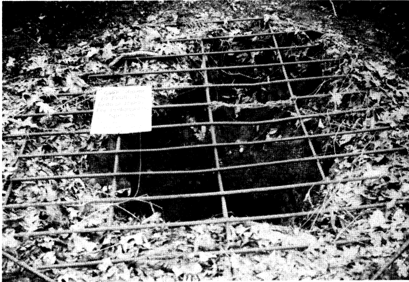
The old entrance gate to the Dry Hole entrance to Turnback Cave in Lawrence County. Note the wire replacement of the missing rebar piece. Because rebar is so easily removed with a hacksaw, rebar gates suffer much damage from vandals.
