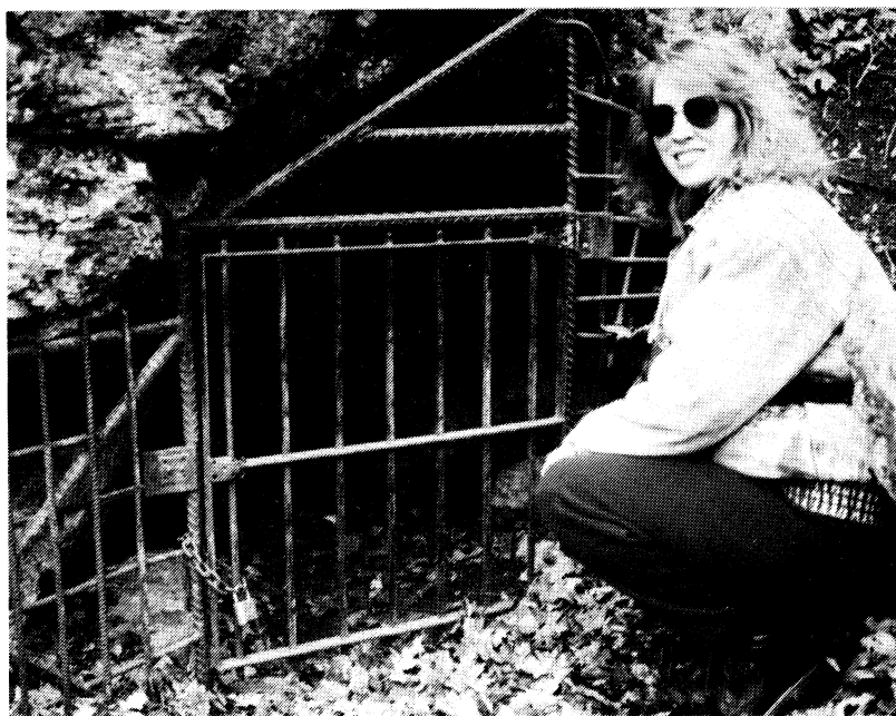
Alicia Beard at the rebar gate to Island Cave in Camden County. To be more bat-friendly, the vertical bars should be 25 inches apart, the spaces between horizontal bars no less than 6 inches wide. To be more vandal-resistant, the rebar should be replaced with angle iron and the locking mechanism should be protected against blows from a hammer, hacksaw or pry bar.
