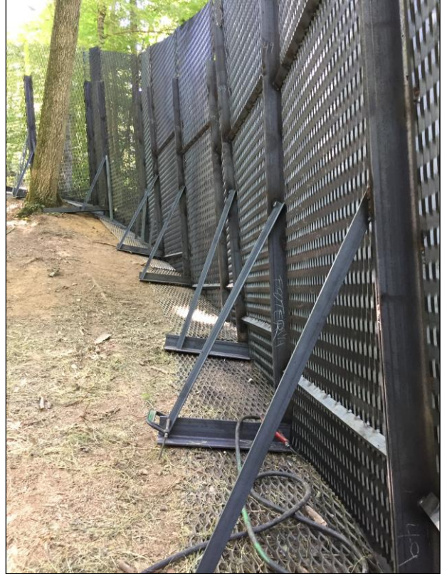
Left and Right: Powers Fence at Tobaccoport Saltpeter Cave during earlier stages of construction, showing details of expanded metal skirting, support footers, inside braces, and horizontal stays. Photos by Jim Kennedy.
