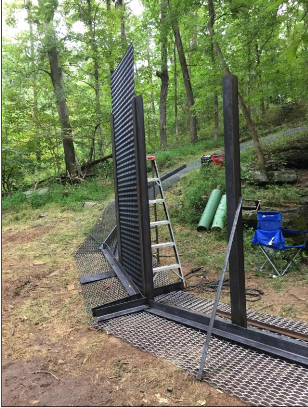
Left and Right: Powers Fence at Tobaccoport Saltpeter Cave during earlier stages of construction, showing details of expanded metal skirting, support footers, inside braces, and horizontal stays. Photos by Jim Kennedy.
